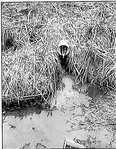
Figure 2: Direct Discharge from a Straight Pipe
